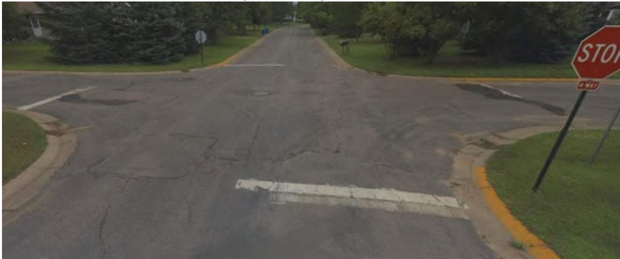
Figure 1: Failing Pavement
